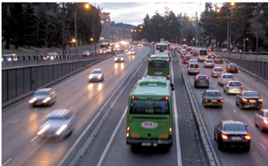
BUS-HOV lane on the A-6
